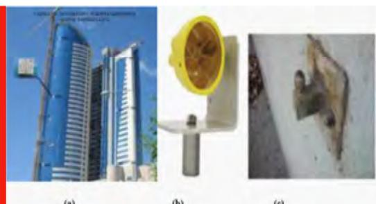
**Fig. 3: Location of the benchmarks on the object (a); Monitoring prism (b) and sedimentary mark (c) Systematical instrumental observations at the geo-monitoring stations mean determination of the benchmarks position in space at a given time with the fixation of the geological factors using the total electronic station Leica TCA 1202.**
