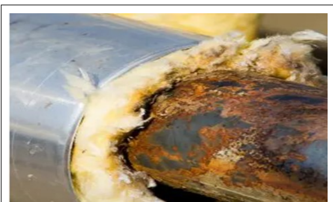
Fig.5. visual test method for corrosion under insulation
