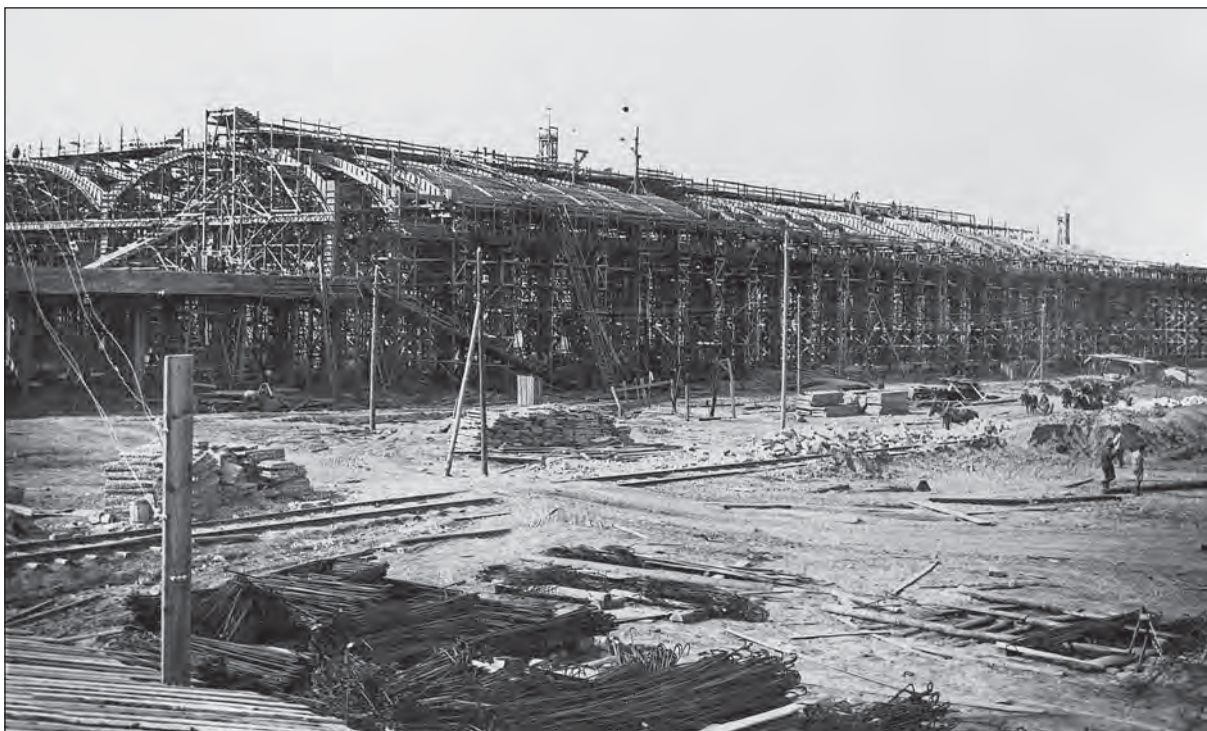
Construction of an aviation plant. Kazan. 1936.
