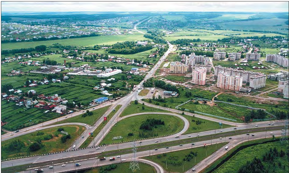
Two-level transport junction. Kazan. 2010.
