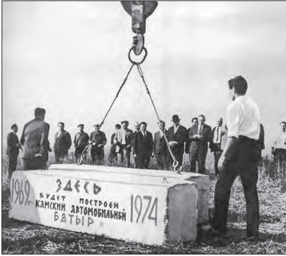
Laying of the first stone of the Kama Automobile Plant. 1969.
