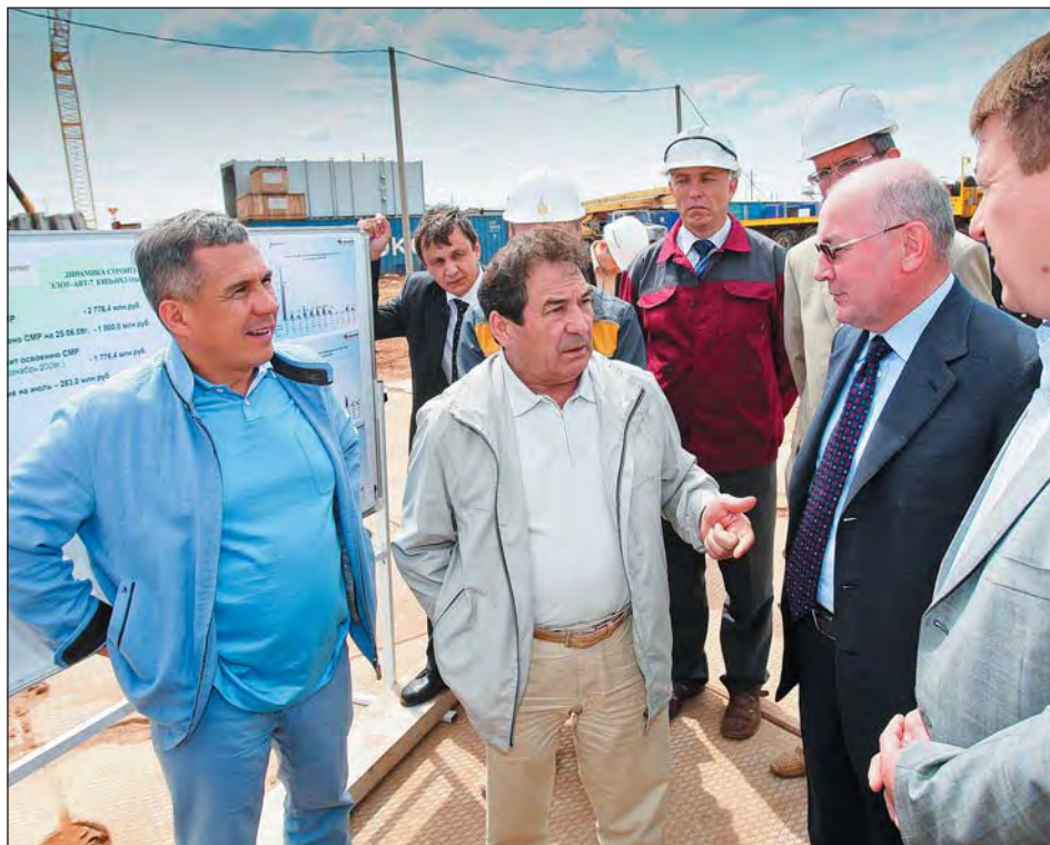
President of the Republic of Tatarstan R. Minnikhanov and CEO of PJSC Tatneft Sh. Takhautdinov at the construction site of PJSC TANEKO. Nizhnekamsk. 2009.
