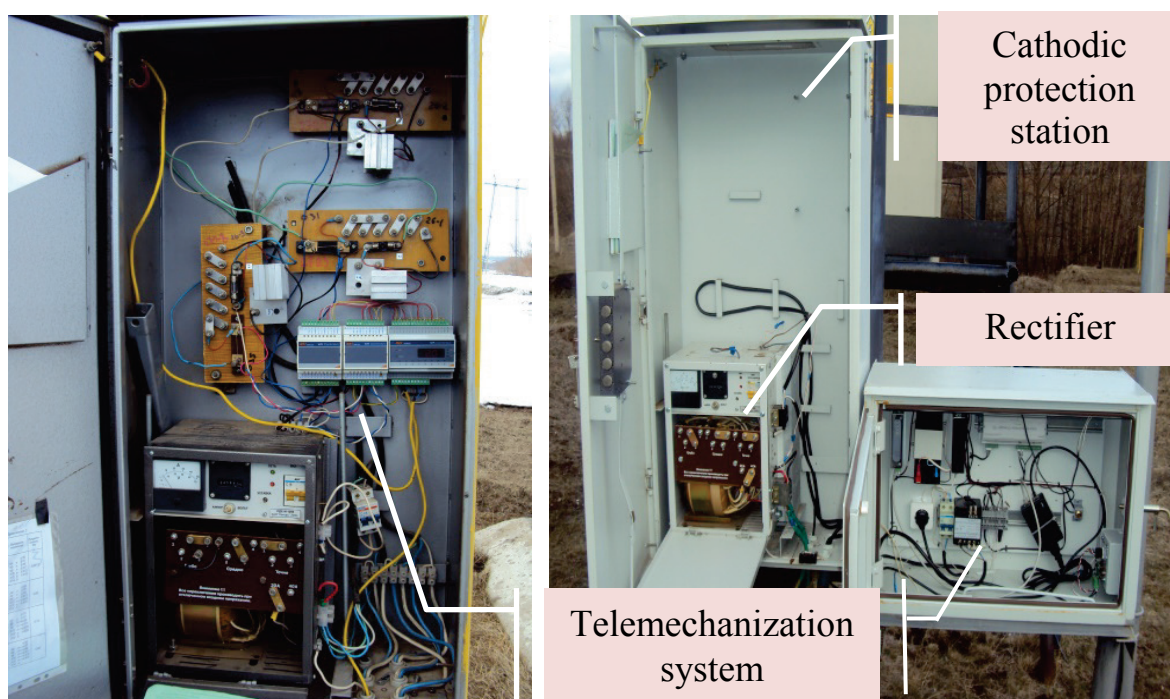
Fig. 6.1. Cathodic protection stations of OGPD Leninogorskneft with the telemeterization system located inside CPS (left) and in a single cabinet (right)
