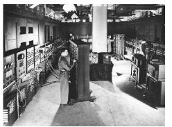
The size of ENIACs numerical "word" was 10 decimal digits, and it could multiply two of these numbers at a rate of 300 per second, by finding the value of each product from a multiplication table stored in its memory. ENIAC was therefore about 1,000 times faster than the previous generation of relay computers. ENIAC used about 1,800 square feet of floor space, and consumed about 180,000 watts of electrical power.
