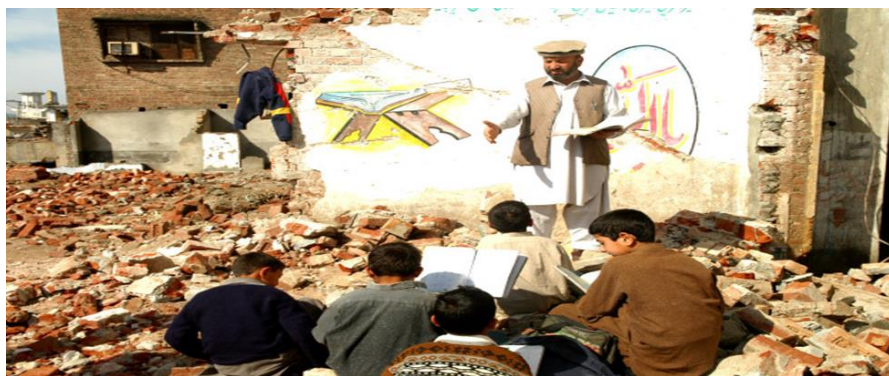
A glimpse on the current condition of the FATA destroyed schools.
